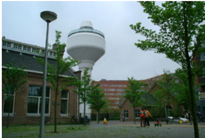
GWL-terrein, Westerpark, A'dam
